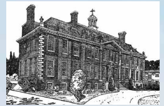
▲ The Cupola and clock as seen on the original Great House
